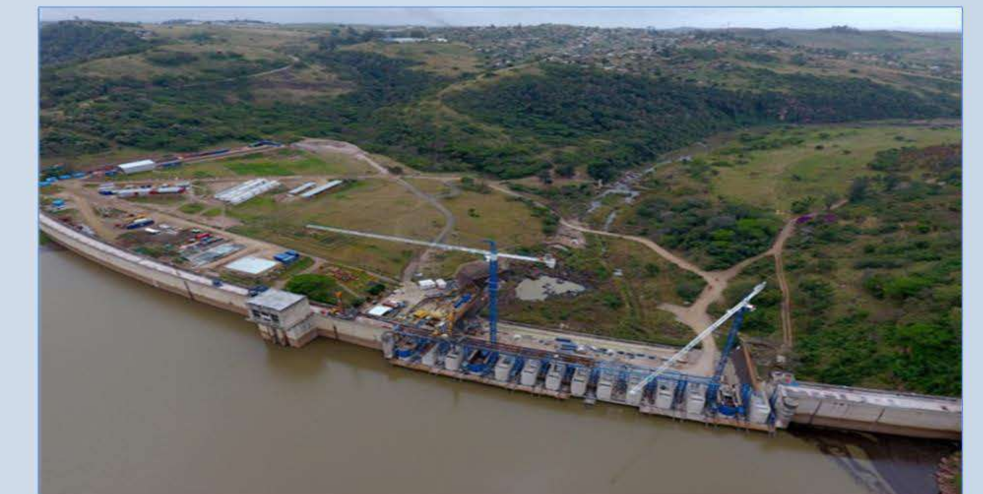
Raising the wall - 2016
